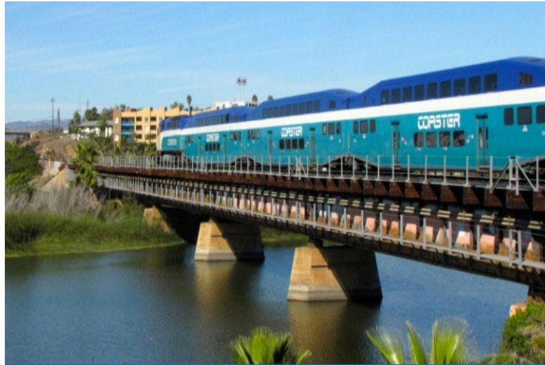
Eastbrook to Shell Double Track
