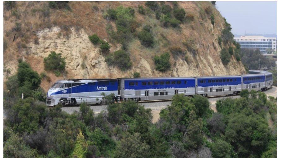
Sorrento to Miramar Double Track Phase 2
